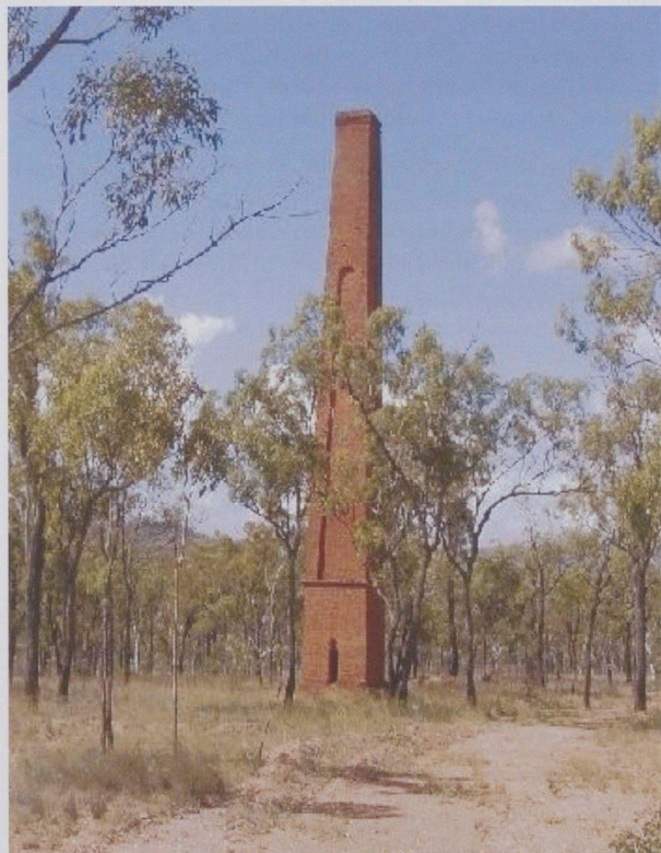
TFTA hazardous site, Argentine smelter.
