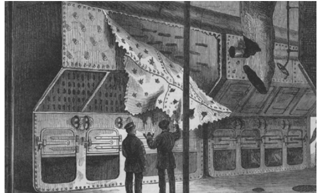
Figure 19. Boiler room damage, HMS Thunderer , July 1876. The accident was ascribed to a faulty safety valve, which killed 15 and injured 70 men, 30 of whom later died. 69 Cerberus 's boilers were generally identical in design (see also Figure 32).
