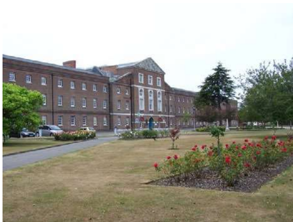
Figure 23. Façade, ex-RNH Haslar, 2009. 65 Having been closed at that time, the site has since been redeveloped for retirement housing. The blue doorway of the main entrance seen here had a rail trolley-way to Haslar Creek (to the right) for receiving patients.
