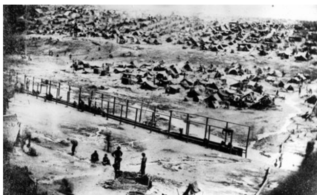
Figure 1: Photo of USA Union Army soldiers at the Andersonville, Georgia prison camp showing the crowded conditions under improvised shelters with field latrines (sinks) in the foreground that led to thousands of prisoner deaths due to gastrointestinal infection. Photo by AJ Riddle in 1864 via the National Parks Service ( https://www.nps.gov/media/photo/gallery-item.htm ). Now in the public domain.
