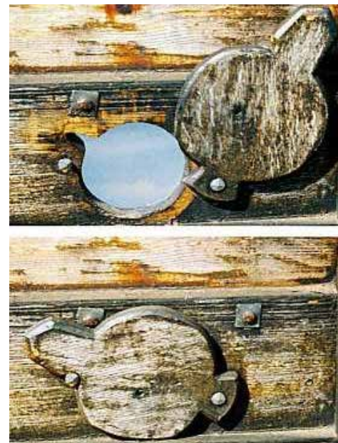
Gokstad ship oar port covers. 42 The port slot at 10 o'clock in the upper photo is for the oar blade.
