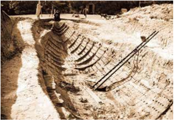
Sutton Hoo ship burial site found 1939, dated c625 CE. 36 Note that, although the wood had not survived, the clinker construction of the hull and the ribs have been preserved in the soil. Also, note the iron rivets.
