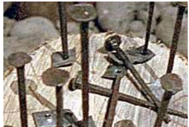
Replica Viking Age iron boat rivets and washers. 35 Each rivet was inserted from the outside of the hull while red-hot so the bottom edge of the uppermost plank or 'strake' overlapped the top edge of the strake below. A washer was placed over each rivet inside the hull and hammered in place.
