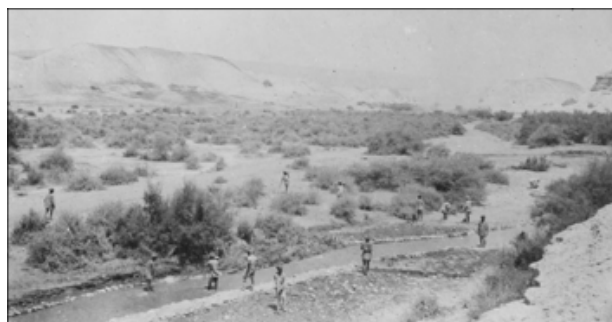
Canalisation of the Wadi el Auja by Sikh pioneers (engineering support troops), lower Jordan valley, 1918. The working party is straightening the stream course and lining the banks with rock. (AWM photograph no. A00328.)
