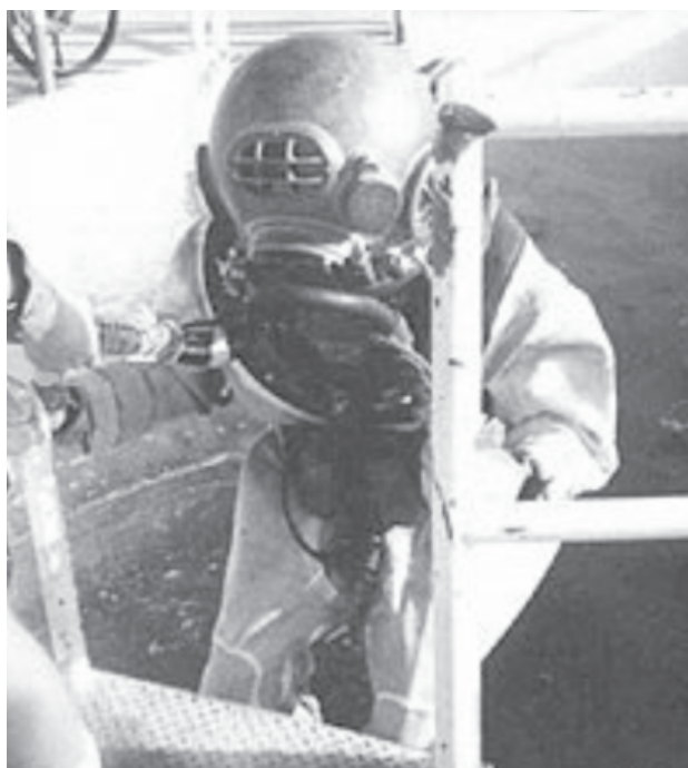
Figure 4. A diver in a Mark IV diving helmet and surface-supplied air, prepares to descend.
